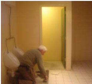
Tiling GAA grounds
