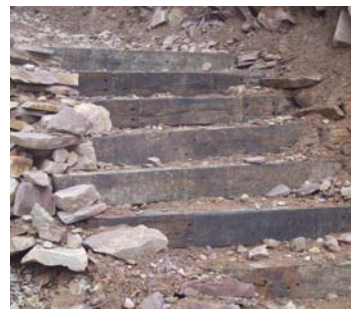
Steps constructed by RSS
