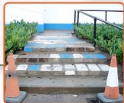
COMPLETION OF STEPS at Killarney Athletic
